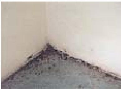
Discoloration is a sign of mould. However, all discoloration is not due to mould. Carpeting near baseboards, for example, can be stained by outdoor pollution entering the home.
