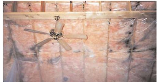
But the mould issues are the same. If there is an exterior leak in an unventilated area, such as an exterior wall, water can accumulate and mould can develop. The mould can eventually cause wood failure, and the result is an expensive renovation project.
