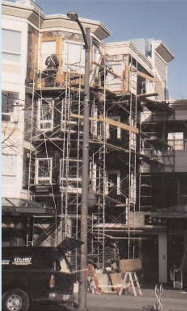
Hundreds of condominium buildings – most constructed during B.C.'s housing boom – are leaking and rotting. Fungi and moulds have grown on floors and walls and water has gotten in everywhere. Conservative estimates say it will take over \$1 billion – most of it from the owners – to repair the leaky, poorly built condominiums in southern British Columbia. Many condominium owners were faced with major structural repairs that devoured retirement savings and rendered their units unsaleable.
